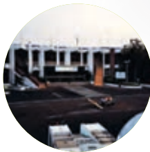
Ambouli International Airport (Djibouti City)
